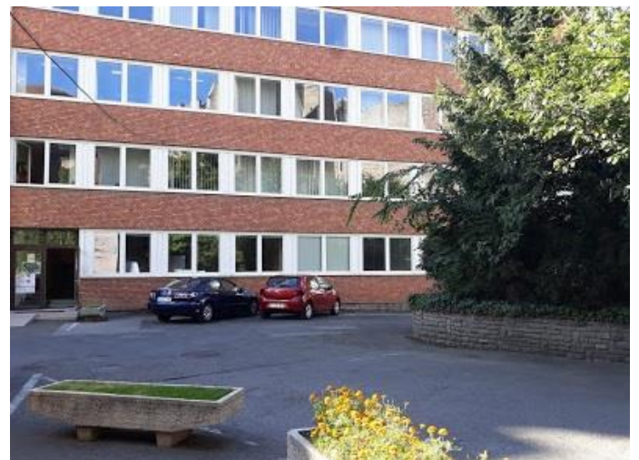
SCHOOL BUILDING ON THE LEFT
